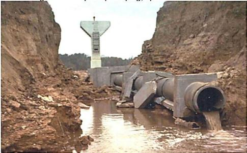
Fonte: RCP Spillway Anti-seep Collars Schnabel Engineering Piping Failure
