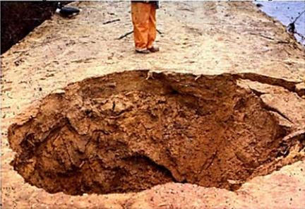
Fonte: Sinkhole in crest of new Dam in Maryland-Piping along Spillway Conduct.
